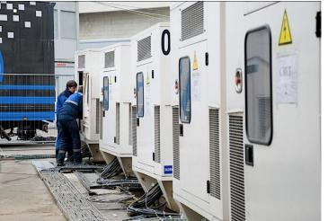
The use of the temporary power supply systems is essential to ensure that television broadcasts, as a main and reservation power source. For example, during the Eurovision-2009 Song Contest in Moscow, were used 27 diesel generating sets with a total capacity of 12.4 MWt.
